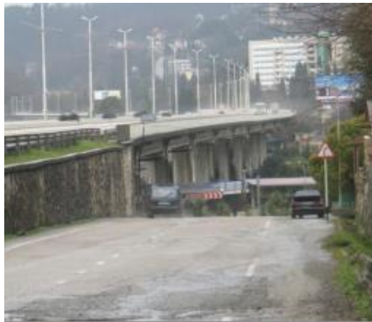
Fig. 3 Electric lighting of roadway on the bridge
