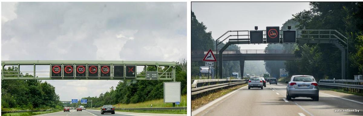
Picture 5. Information construction of the beam and frame system
